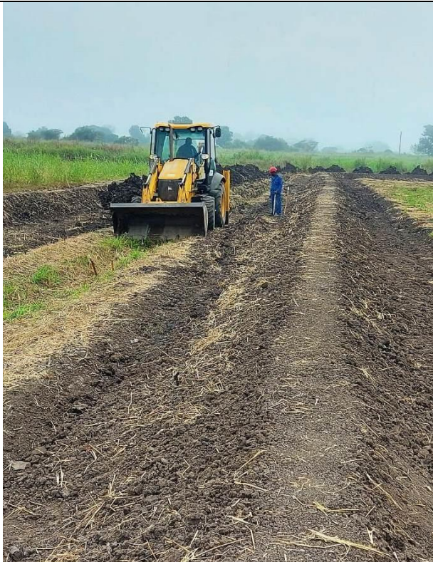
Foto 19: JCB machine excavating the field drains
